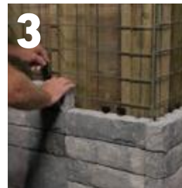
3 Attach Tandem Veneer with Connector
